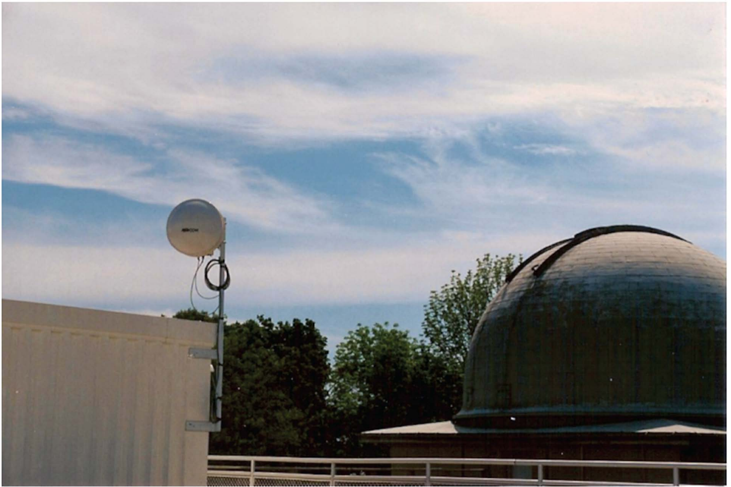
Early 10 Mbps Fixed Wireless Installation at MIT, Cambridge, 1989 by Microwave Bypass Systems, Inc.
